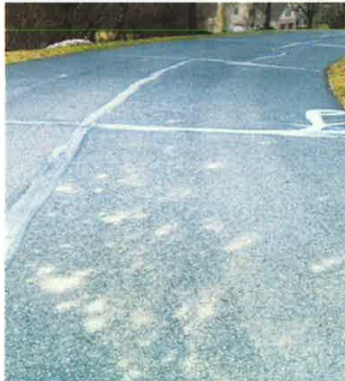
Hawk Road (One of several Roads Crack Sealed)
